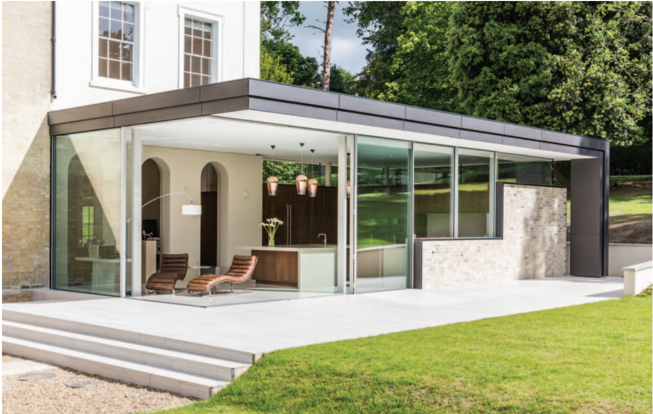
The addition of this spacious, contemporary extension to a magnificent listed Georgian mansion incorporating Fusion Vista 19 at different levels with a fully opening corner
