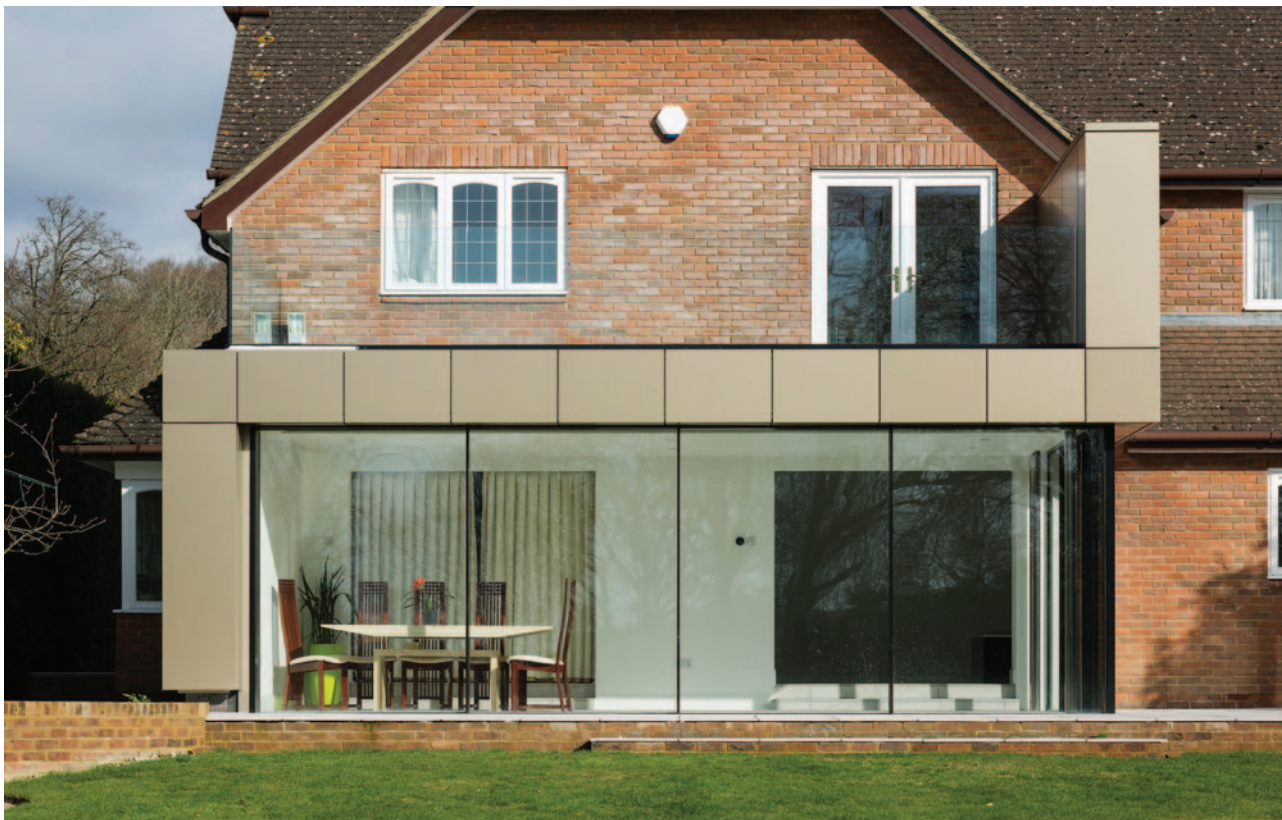
This impressive glazed extension incorporating a four track Fusion Vista 19 system with a fully opening corner was a retirement gift from a 'loving husband to his wife'.
